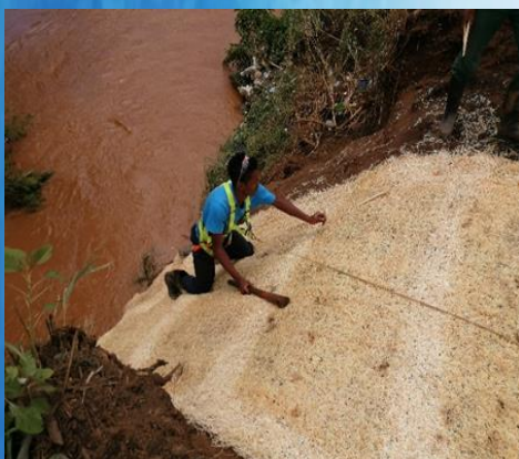
Figure 1: Andile installing pegs on the RECP's that prevents soil erosion
